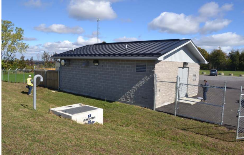
View of Water Booster Pumping Station building post construction.
